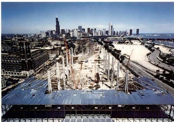
Fast-track public-sector exhibition hall construction over live rail.
