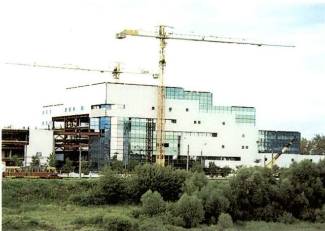
Prefab Nordicon facades (Finland) accelerate Russian construction.
