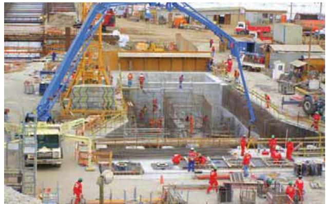
SEA WATER TANK, IMPERMEABILIZADO CON PRODUCTO PENETRON.
