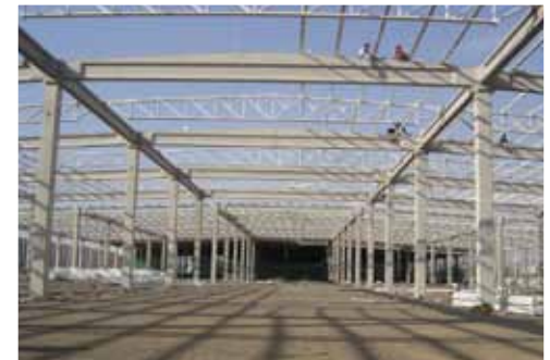
NAVE INDUSTRIAL BODEFLEX 33.750 m 2
