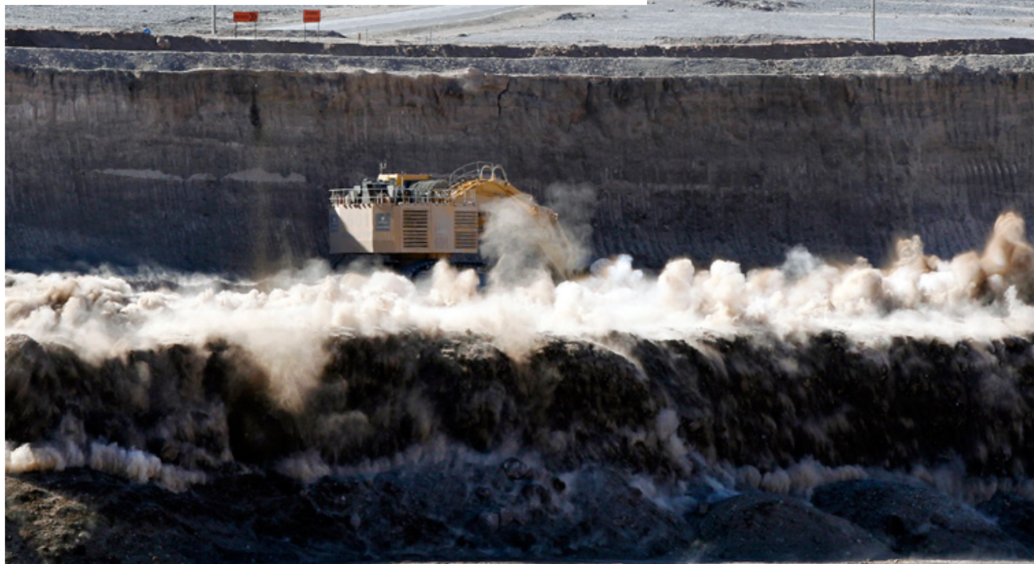
End of pre-stripping, 228 million tons of sterile material had to be removed, the equivalent of 70 times the Santa Lucía Hill in Santiago. Courtesy of Codelco.
