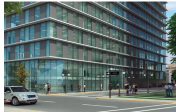
LEED® GOLD CS v2009 - Core and Shell
