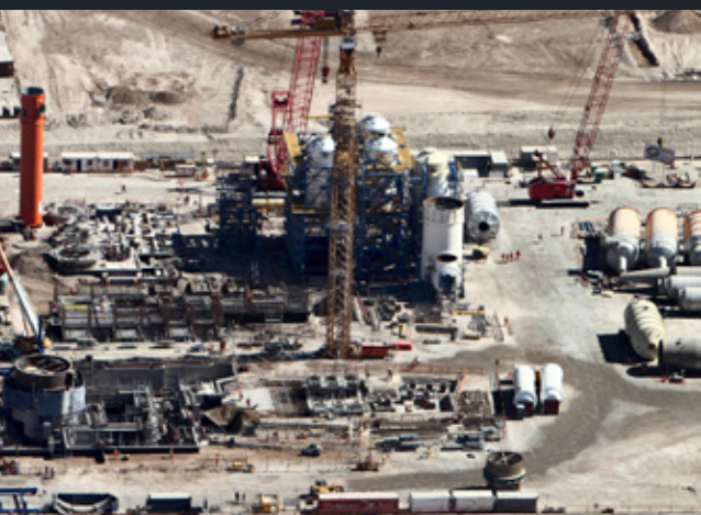
In area 5000 corresponding to the roasting site, calcine hopper buildings were considered, pressurized vessels for pneumatic transport, ecometals, compressors room and two electric rooms. Courtesy of Codelco.
