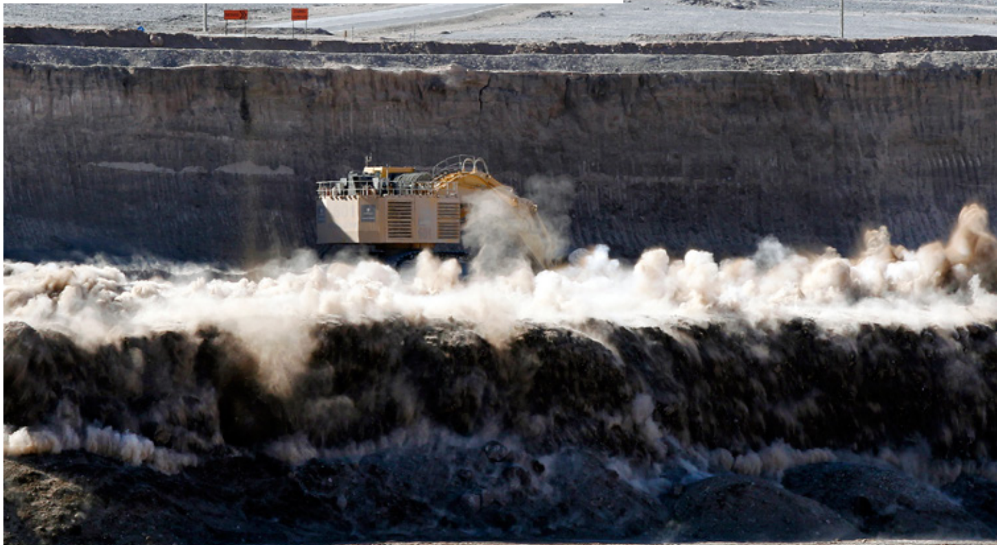
End of pre-stripping, 228 million tons of sterile material had to be removed, the equivalent of 70 times the Santa Lucía Hill in Santiago. Courtesy of Codelco.
